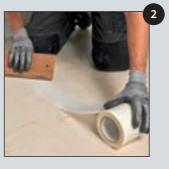
Mark out the position of the Modul'up sheets on the subfloor. Apply the Modul'up adhesive tape, non-slip side down, along the marked joins and along door threshholds.
