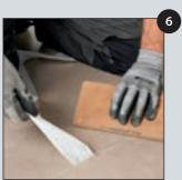
Once completed, simply press down on the joint to improve adherence between the floor covering and the Modul'up adhesive tape.
