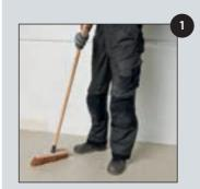
Brush or vacuum the subfloor. In case of a new substrate, apply a primer.
