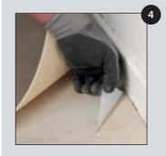
Trim around the edges, but avoid cutting in too tightly (leave a gap of 1mm). Skirting can be fitted for a more aesthetic finish.
