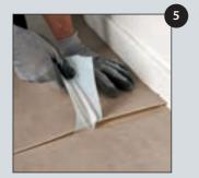
Peel away the protective film (tearproof) while remaining as close as possible to the covering and allow the edges to fall back down.
