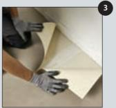
The tape must be positioned so that both sheets cover the tape. Place the floor covering in the room, so that it covers the entire surface and laps up slightly along the walls (+10 cm).
